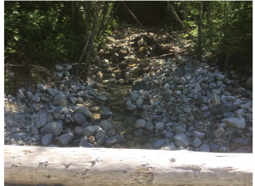
Upstream from Crossing
