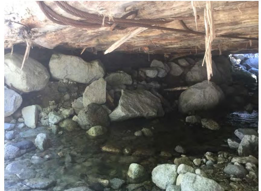
Right Bank Abutment when facing downstream
