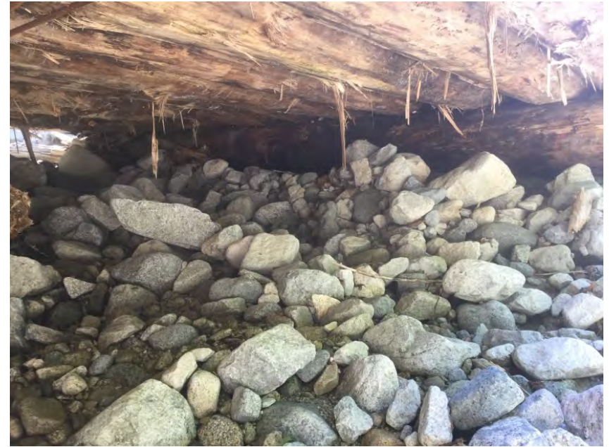
Left Bank Abutment when facing downstream
