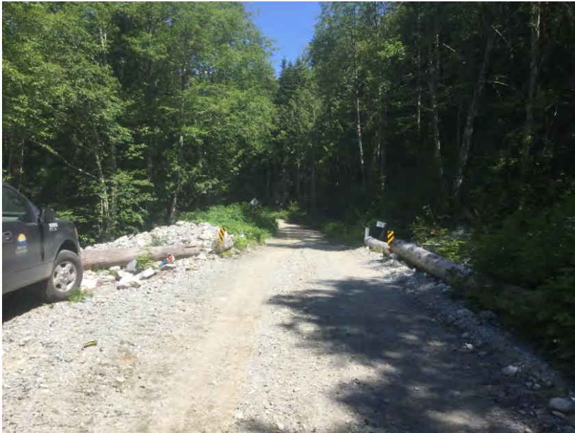
Approach from Left Bank when facing downstream
